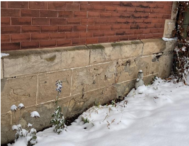
Plate 14: Parged stone foundation
