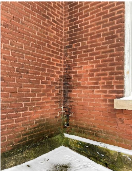
Plate 26: Location of former downspout on east elevation
