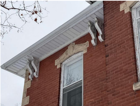
Plate 12: Overhanging eaves and paired bracket detail
